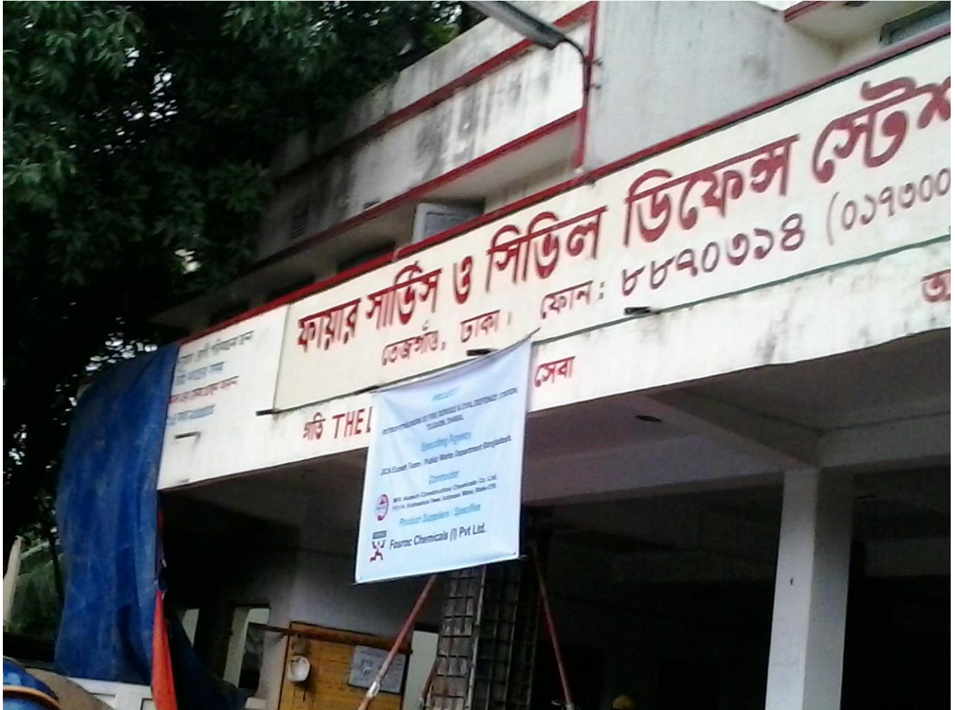
Fig: Fire Brigade Building
