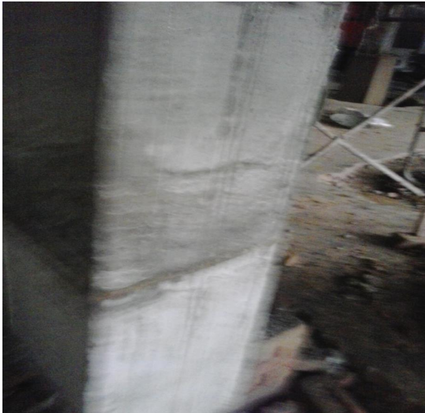
Fig: Column After Micro Concrete Encasement
