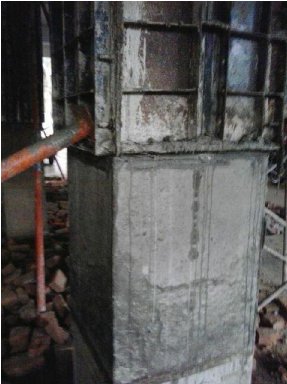
Fig: Column after Micro Concrete Encasement
